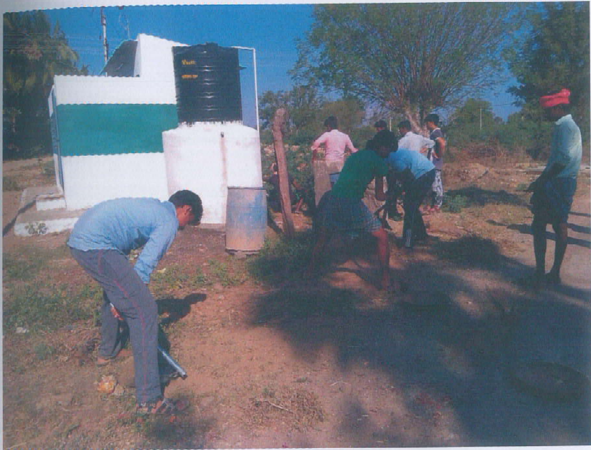
They cleaned under the over tank
